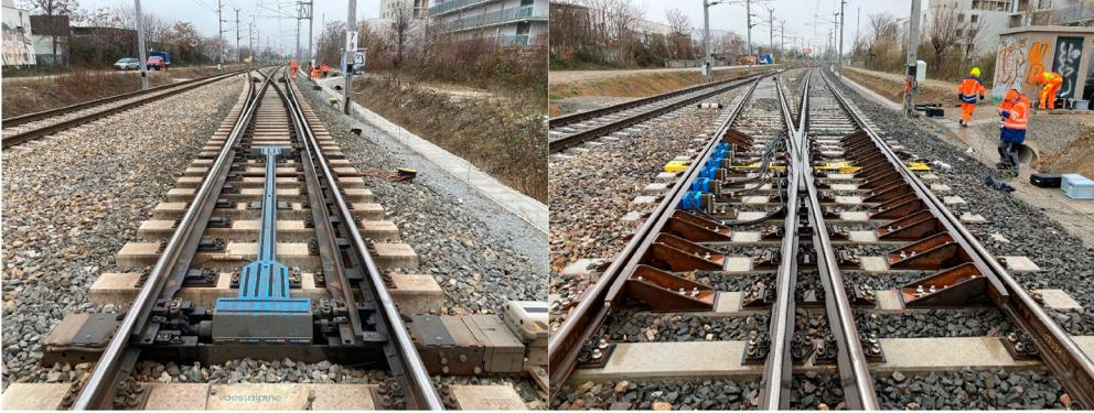
**Figure 1.** Pictures from the demonstrator test site taken by voestalpine Railway Systems GmbH. The whole S&C seen from the switch panel side (left) and detail of the crossing panel (right). Through route to the right and diverging route to the left in both pictures.
